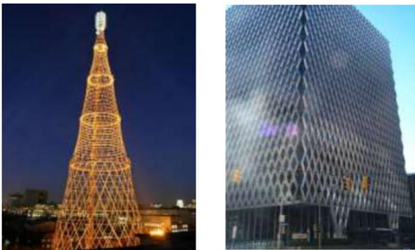
(a) Shukhov Tower in Moscow (b) IBM Building in Pittsburgh
